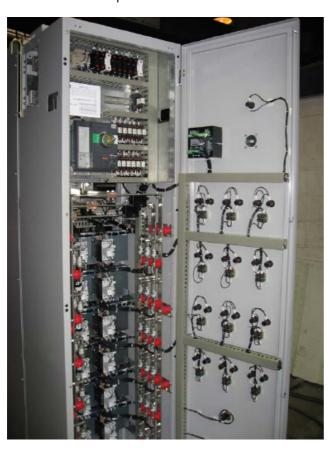
Power Factor Correction equipment supplied to major UK food factory. Panel includes controller, capacitors, contactors, stage fuses, detuning reactors, door interlocked isolator, thermal management, fans and alarms.
