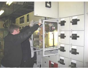
Note that ExEllison Switchgear Services Ltd does not install an ACB into an existing ACB chassis. There is little point in replacing an ACB whilst still relying on aged contact finger clusters. We take the old ACB out completely right back to the basic connections. This weak point is removed to ensure the integrity of the new assembly.
