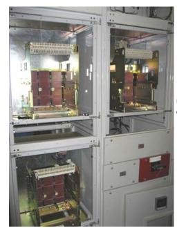
Internal shrouding is fitted to make the ACB module complete. A fully shuttered Cassette is used to ensure the operators safety.
