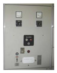
The main LV switchboard was some 20 years old and utilised Ellison GEA air circuit breakers. Whilst the ACBs had given years of good service they had encountered a number of problems with difficulty in closing and failure of the CPR Overcurrent relay fitted. There were also considerations made as to the problems in the supply of spare components in the event of future problems.
