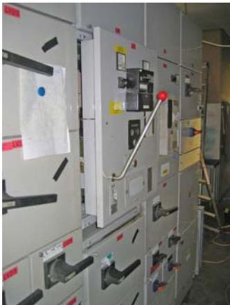
The main LV switchboard was some 15 years old and utilised Ellison GEA air circuit breakers. Whilst the ACBs had given years of good service they had encountered a number of problems with difficulty in closing and failure of the CPR relay fitted. There were also considerations made as to the problems in the supply of spare components in the event of future problems.
