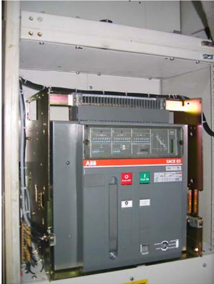
Internal shrouding is fitted to make the ACB module complete. A fully shuttered Cassette is used to ensure the operators safety.
