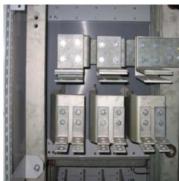
Note that [ExEllison Switchgear Services Ltd](#) does not install an ACB into an existing ACB chassis. There is little point in replacing an ACB whilst still relying on aged contact finger clusters. We take the old ACB out completely right back to the basic connections. This weak point is removed to ensure the integrity of the new assembly.
